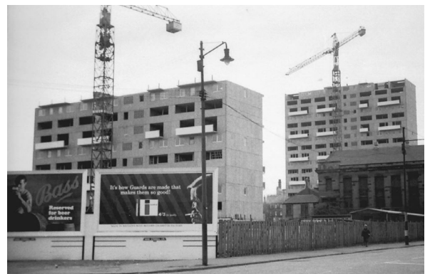
Woodside Multi-storey Towers - Under construction (1960's)
